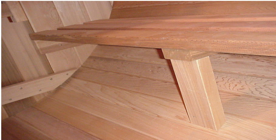
Figure 5 - Seat Installation
